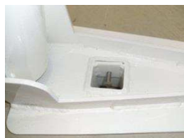
3/8" bolt inside anchor sleeve
